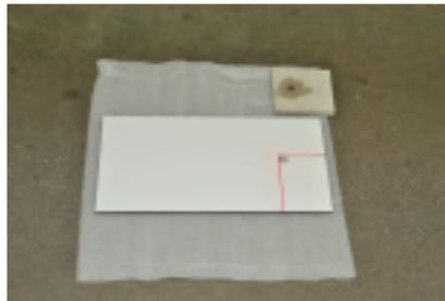
Visually align the template with the pilot hole and finish drilling from the front side.
