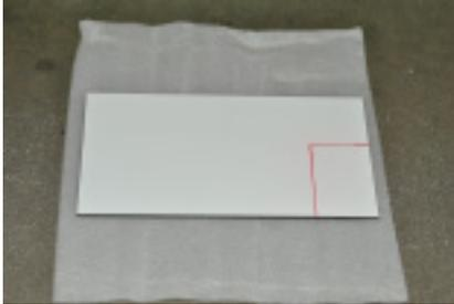
Using a wet core diamond bit and a template, drill a pilot hole, at the inside corner, half way through the tile thickness. Use the template to stabilize the core bit and prevent "walking" and liberally apply water during drilling. Starting to drill from the backside will help minimize chipping of the decorative coating.
